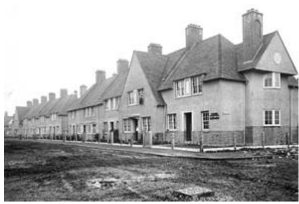
Fig. 12: Fitzneal St showing Clerk of Works office, 1912. (LMA ref: SC/PHL/02/0839)
