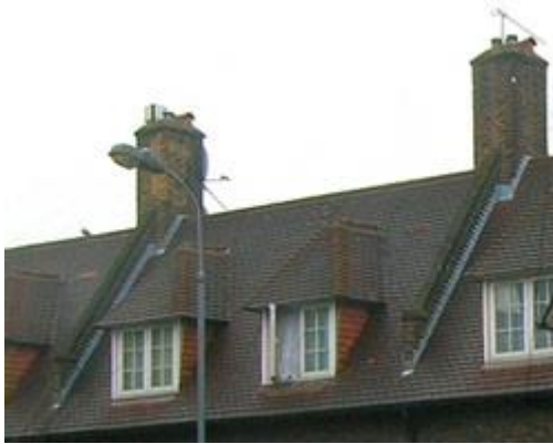
Fig. 13: Close-up of typical extended party walls.
