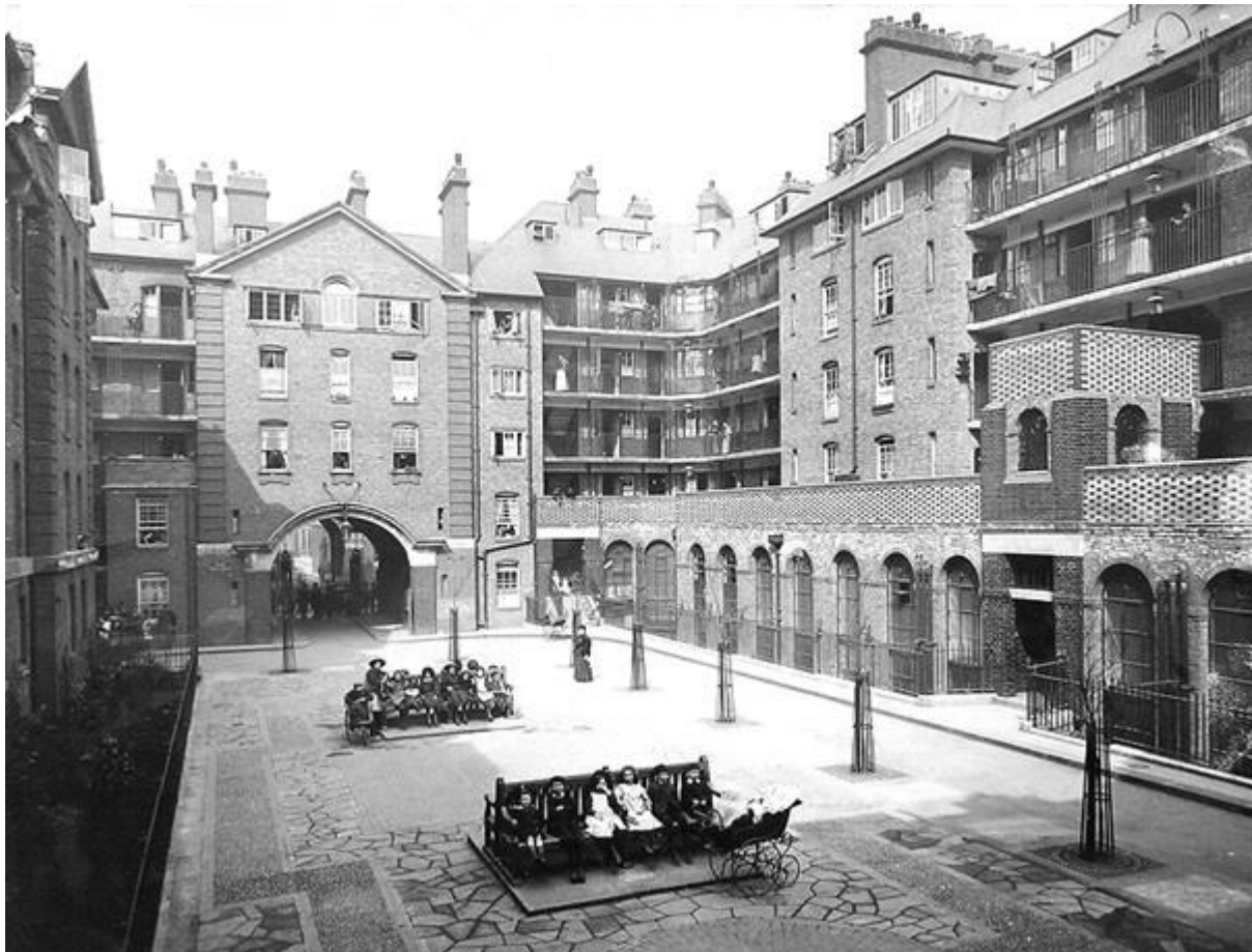
Fig. 5: Laney Buildings (right), 1909 (LMA ref: SC/PHL/02/0769)
