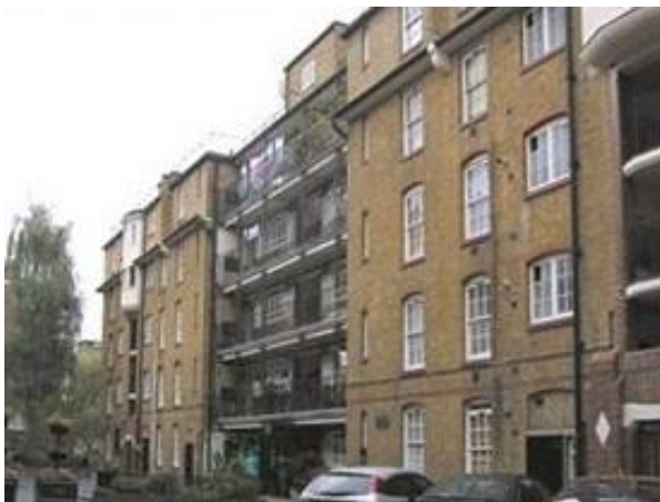
Fig. 9: Buckridge House front, 2009
