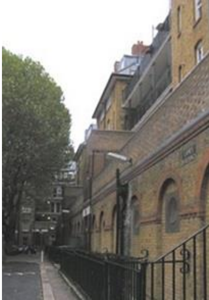
Fig. 11: Laney House, 2009. Windows at rear of shops bricked in
