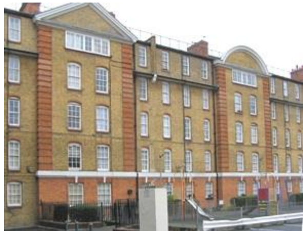
Fig. 10: Buckridge House rear, 2009
