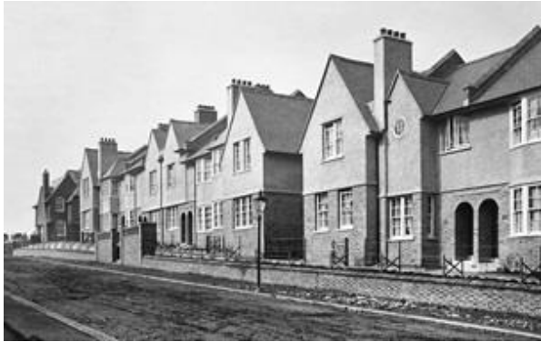
Fig. 7: Norbury Estate, Northborough Rd, 1908 (LMA ref: SC/PHL/02/0835)
