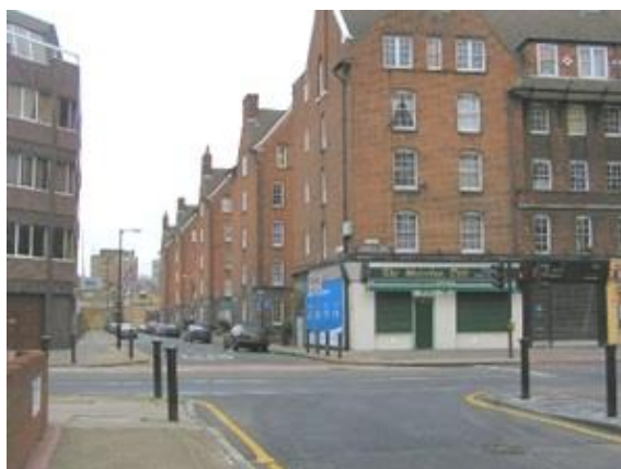
Fig. 7: View down Webber Row showing the ends of the blocks, 2007
