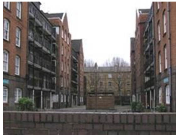
Fig. 6: Webber Row blocks facing each other looking over the yard, 2007
