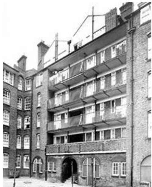
Fig. 5: Rear of Mallory Buildings, 1970 (LMA ref: SC/PHL/02/0829)
