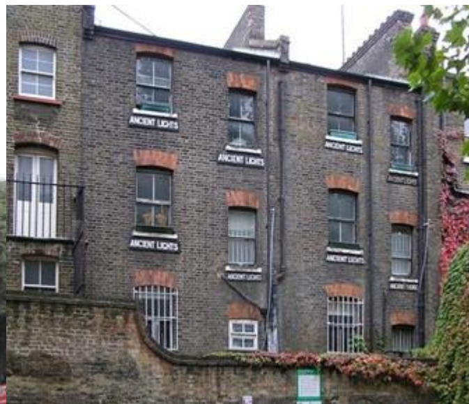
Fig. 7: Adjacent to the rear of Mallory Buildings, 2009
