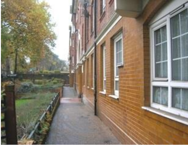
Fig. 8: Detail of the light glazed brick at the front, 2009
