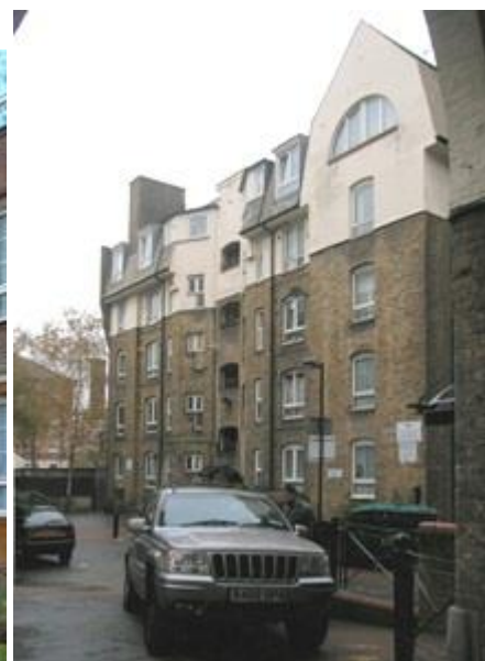
Fig. 7: One of the rear blocks of Renton House, 2009
