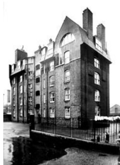
Fig. 4: One of the rear blocks of Briscoe Buildings, 1907 (LMA ref: SC/PHL/02/775)
