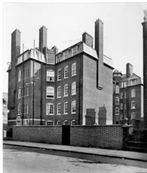
Fig. 7: Bearcroft Buildings rear view (LMA ref: SC/PHL/02/0766)
