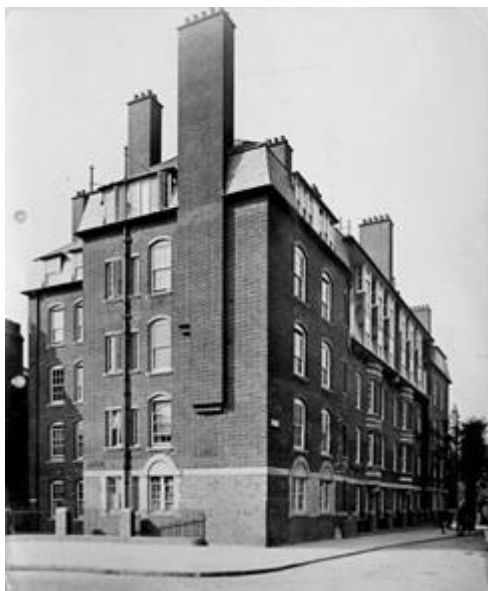
Fig. 6: Bearcroft Buildings front view (LMA ref: SC/PHL/02/0766)
