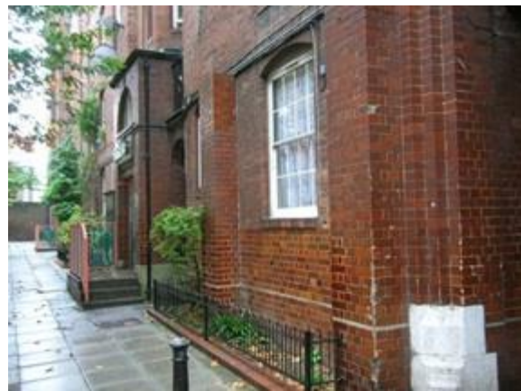
Fig. 11: Detail of glazed bricks
