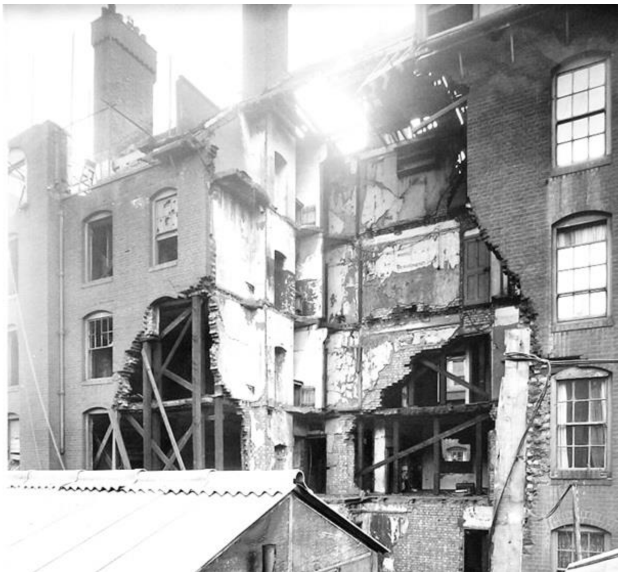
Fig. 7: WW2 bomb damage (LMA ref: SC/PHL/02/0890)
