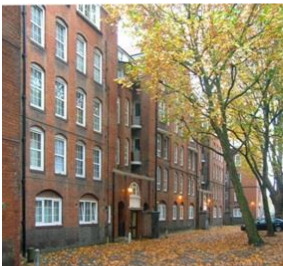
Fig. 9: Wetherbury House, rear, 2009
