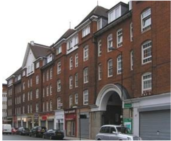
Fig. 14: Chadworth House (from Lever St) 2009
