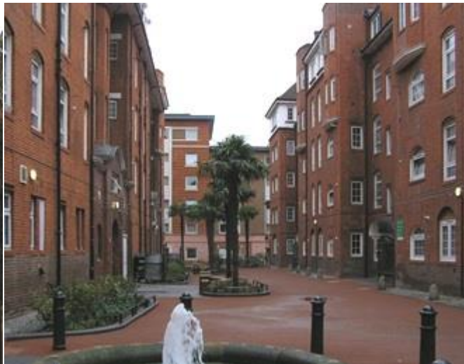
Fig. 16: Chadworth House courtyard 2009
