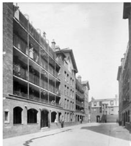
Fig. 8: Wenlake Buildings front with Priestley House on the right (LMA ref: SC/PHL/02/0890)
