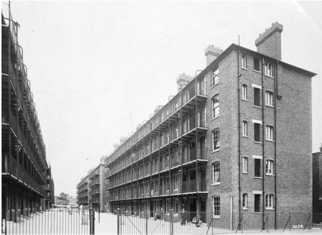
Fig. 3: Preston's Road site with Ontario Buildings in the foreground (LMA ref: SC/PHL/02/0847) Both the blocks and the cottages were erected by Messrs F. & T. Thorne. The sequence of opening was: Ottawa and Baffin, March 1904; Hudson in July 1904; Ontario in August 1904; and Winnipeg and Quebec in September 1904. The cottages were completed in July 1904.
