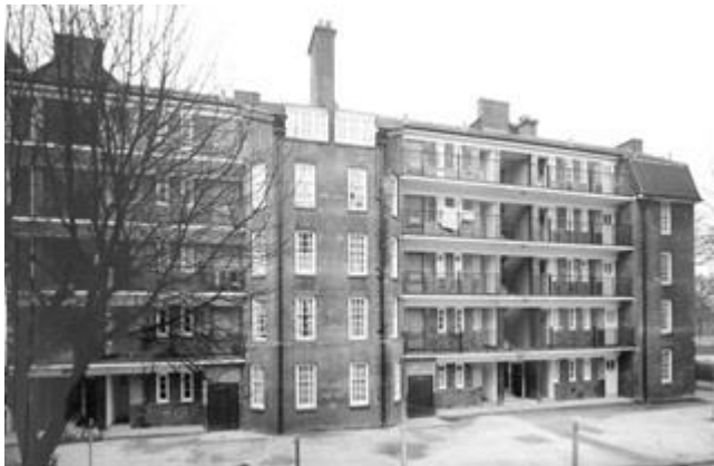
Fig. 10: Walkways of Darcy Buildings facing away from London Fields, 1966 (LMA ref: SC/PHL/02/0885)
