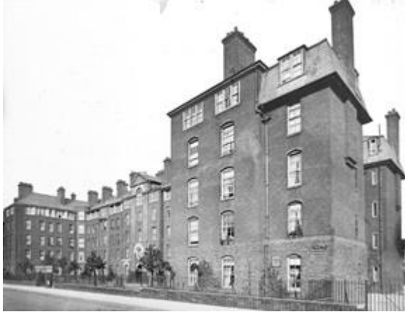
Fig. 8: Front view of Valette Buildings, 1907 (LMA ref: SC/PHL/02/0883)
