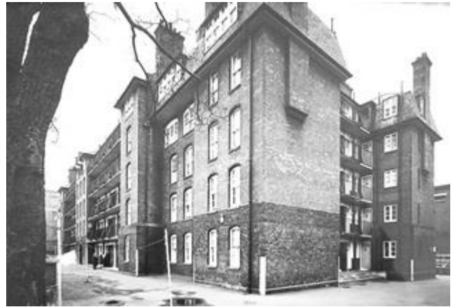
Fig. 9: Rear view of Valette Buildings, 1960s (LMA ref: SC/PHL/02/0883)
