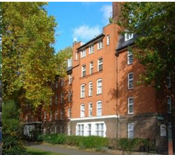
Fig. 13: Rear of Darcy Buildings looking onto London Fields, 2009
