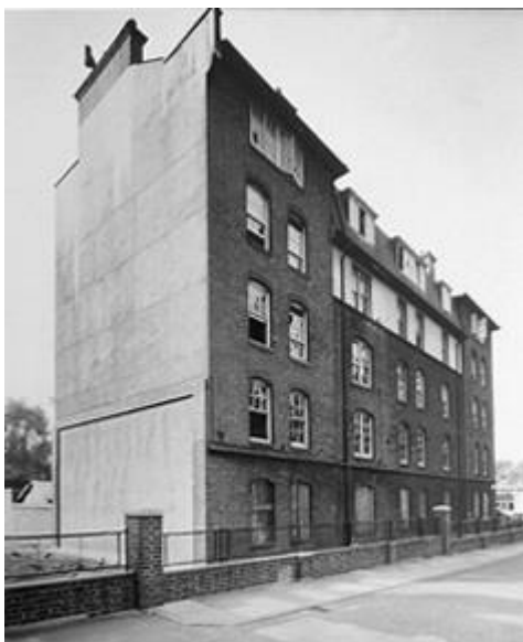
Fig. 2: Benbow Bldgs before renovation, 1960s. (LMA ref: SC/PHL/02/0813)
