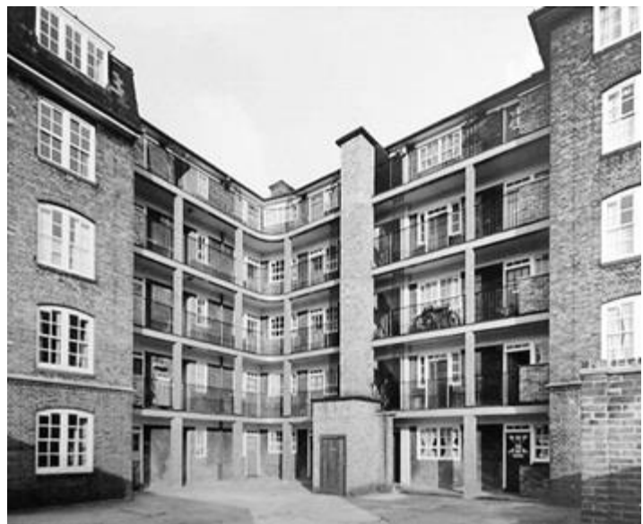
Fig. 3: rear of Benbow Buildings post renovation (LMA ref: SC/PHL/02/0813)
