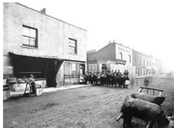
Fig. 9: Swan Lane and Railway Ave, 1903 (LMA ref: SC/PHL/01/040)
