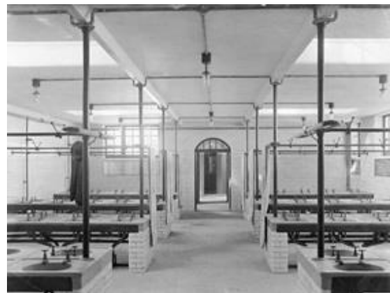
Fig. 10: Carrington House wash room (LMA ref: LCC/AR/HS/02/1044)
