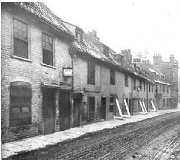
Fig. 4: Mill Lane housing, looking south. (LMA ref: SC/PHL/01/075)
