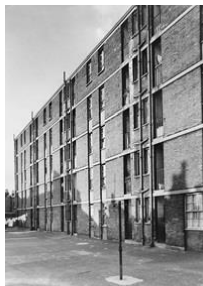
Fig. 7: Rear of Sydney Buildings in the 1960s (LMA ref: SC/PHL/02/0749)
