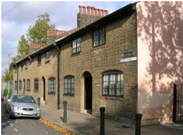
Fig. 5: Hardy Cottages facing Eastney St, 2009
