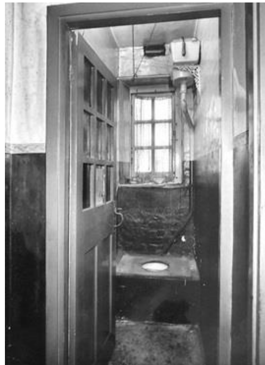
Fig. 9: WC from one of the Millbank Buildings in 1960 (LMA ref: SC/PHL/02/0832)
