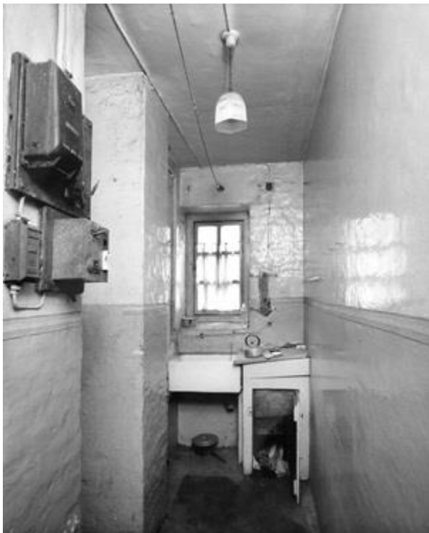
Fig. 8: Scullery from one of the Millbank Buildings in 1960 (LMA ref: SC/PHL/02/0832)
