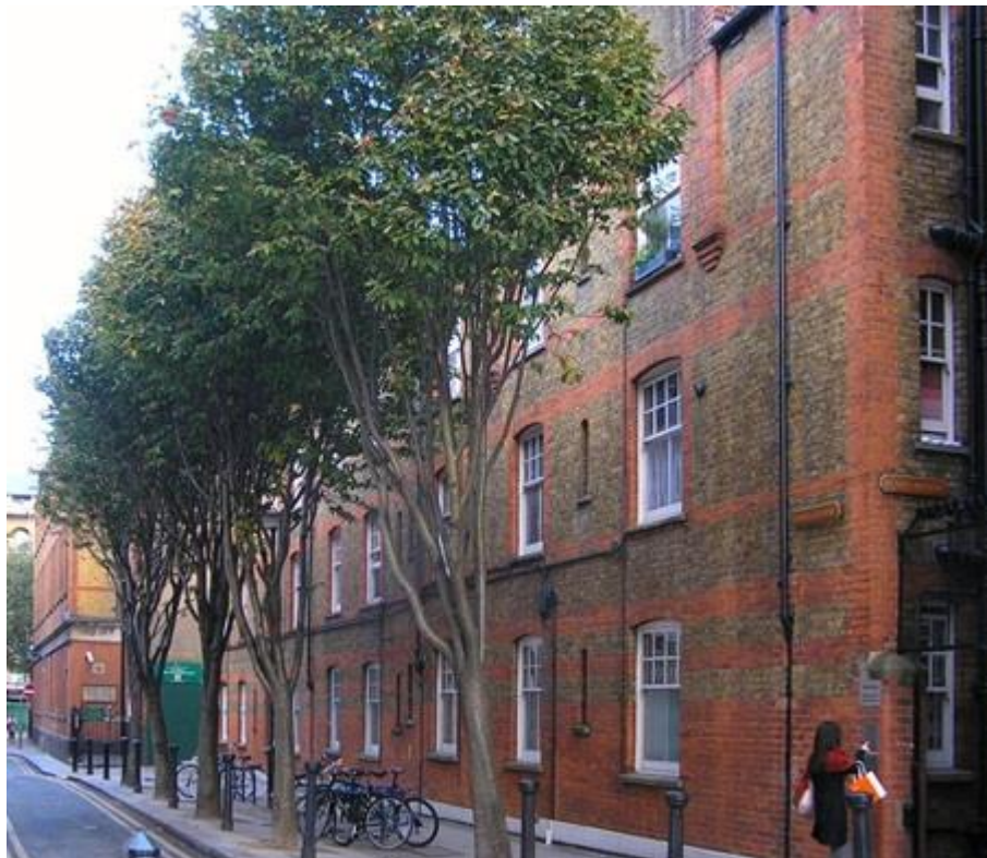
Fig. 9: Powis House, Macklin Street, 2009
