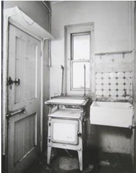
Fig. 5: Scullery of Dellow Buildings taken before renovation in 1960 (LMA ref: SC/PHL/02/0778)
