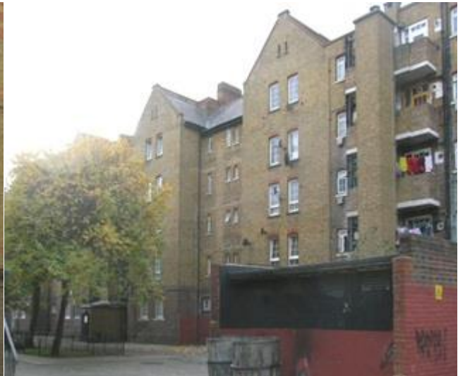
Fig. 8: Dellow House, rear, 2009
