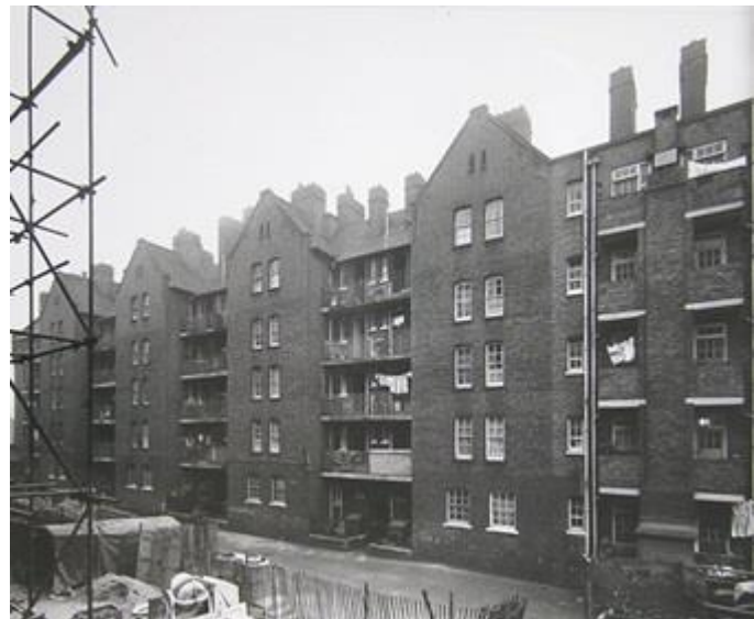
Fig. 4: Rear of Dellow Buildings during modernisation (LMA ref: SC/PHL/02/0778)
