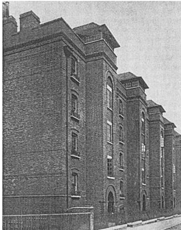
Fig. 1: Council Buildings, date unknown
