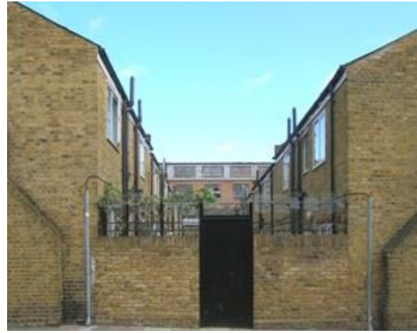
Fig. 7: Cranford Cottages yard entrance, 2009
